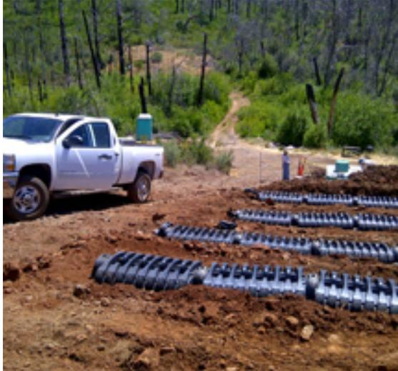
As with the half-pipe design, the chamber protects the trench and helps distribute the effluent evenly over the trench bottom just below the ground surface where biological activity is greatest. Effluent infiltrates the native soil surface and percolates down through underlying soil where additional nutrient and pathogen removal occurs.
