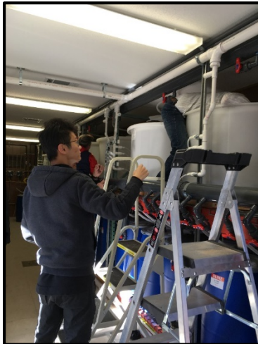
Staff Installing Media into Sand Filters
